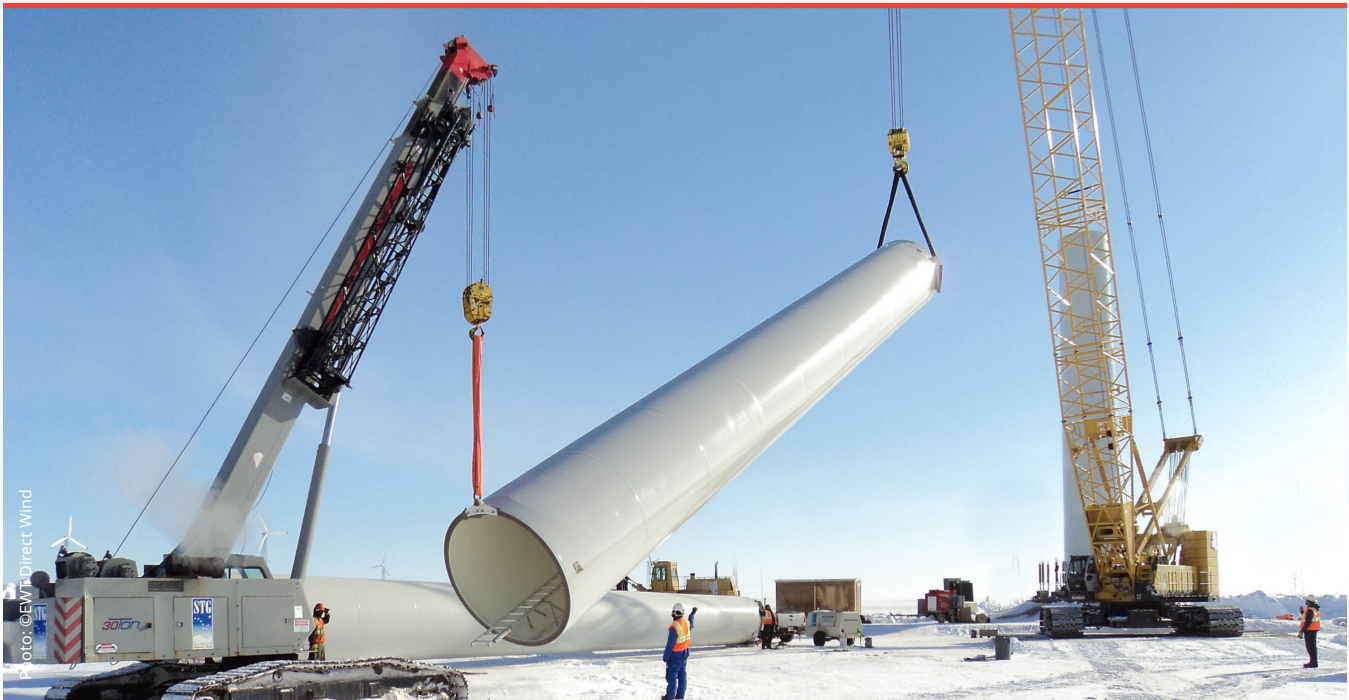
Northern wind turbine construction
