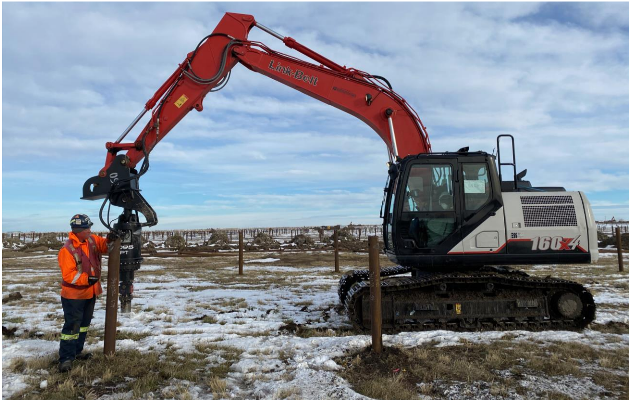
Pilings being installed at Claresholm solar project
