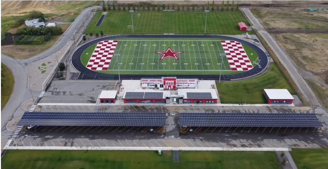
Solar panels cover parking stalls at Raymond football stadium
