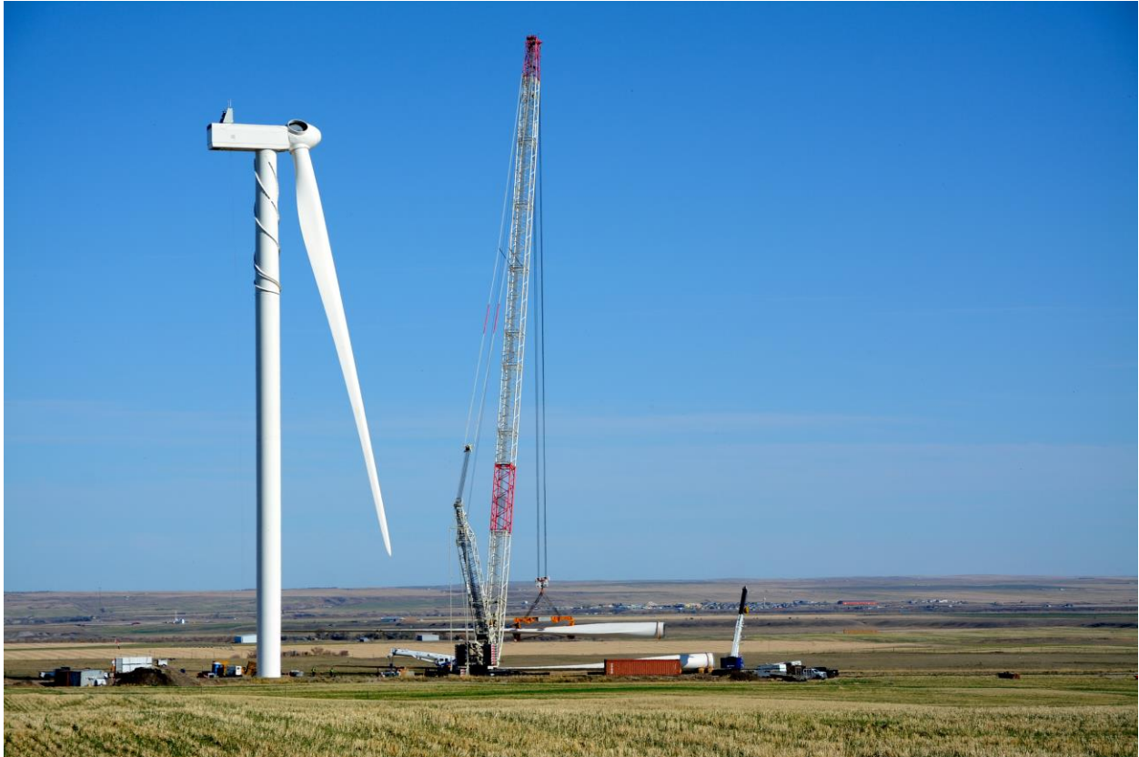
Wind turbine construction in Southern Alberta
