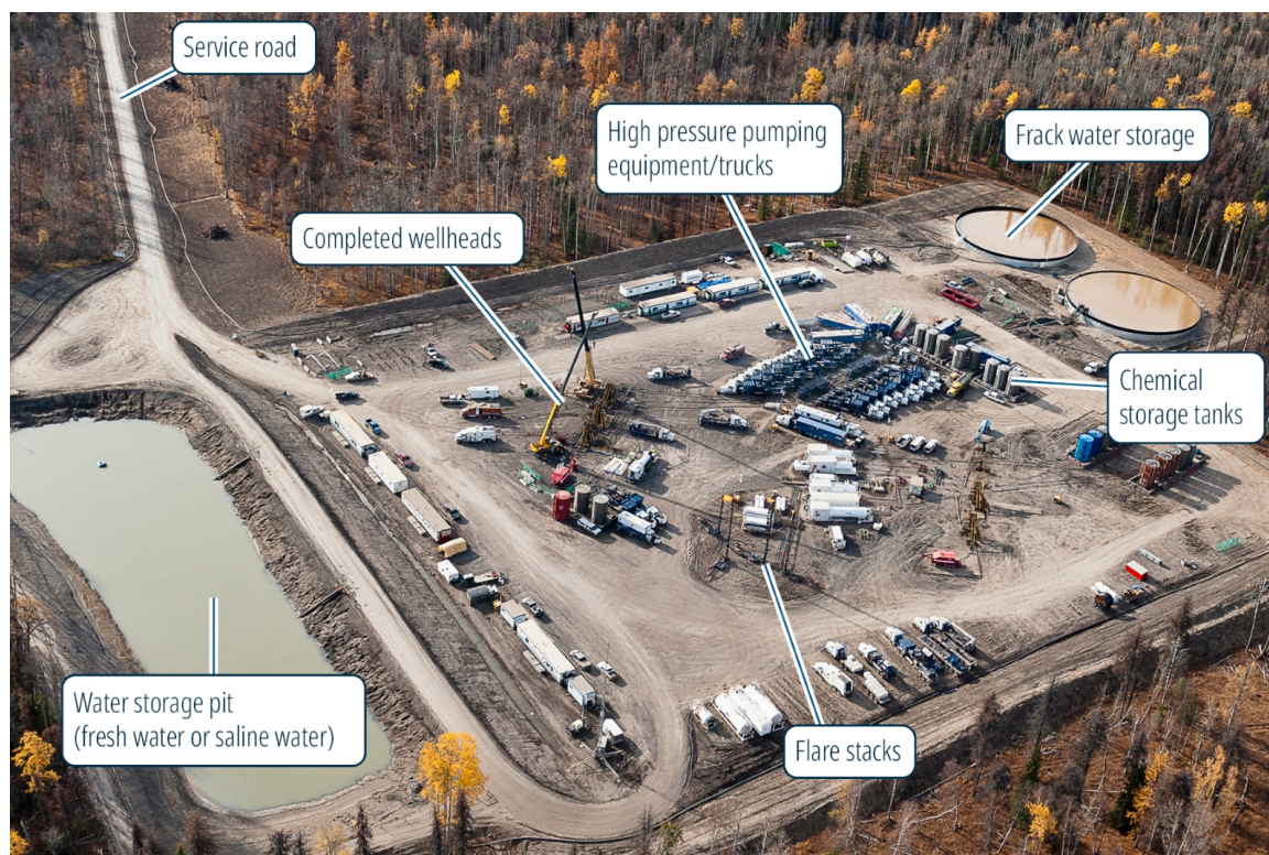
Figure 5. Hydraulic fracturing site
