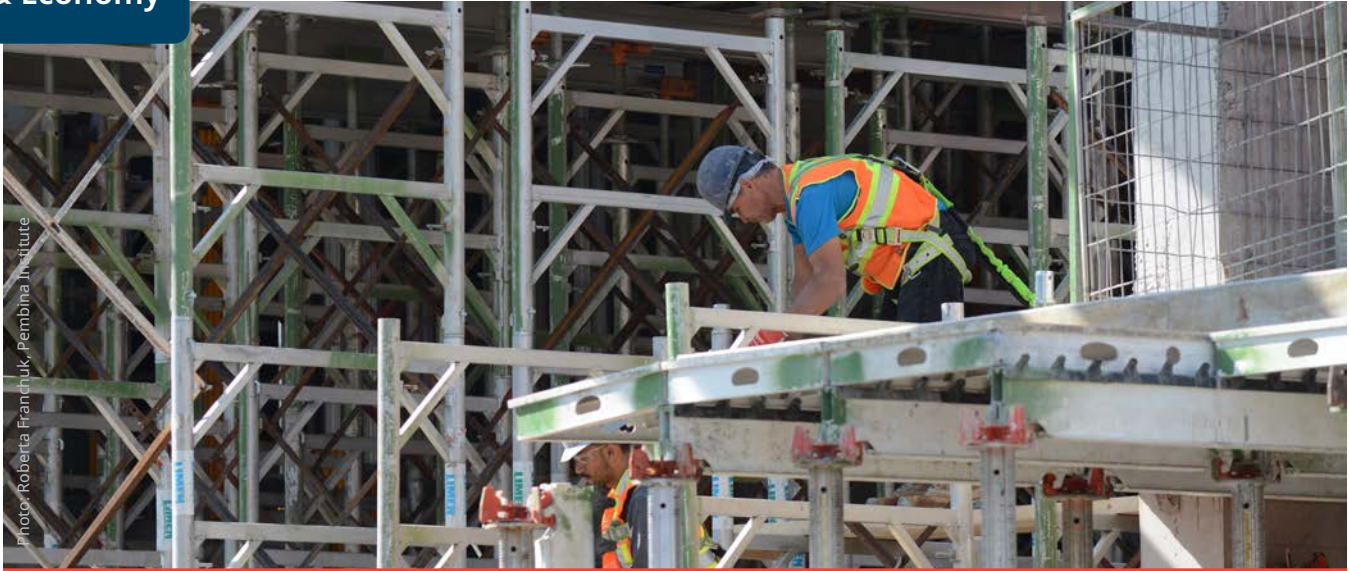
Construction in Toronto
