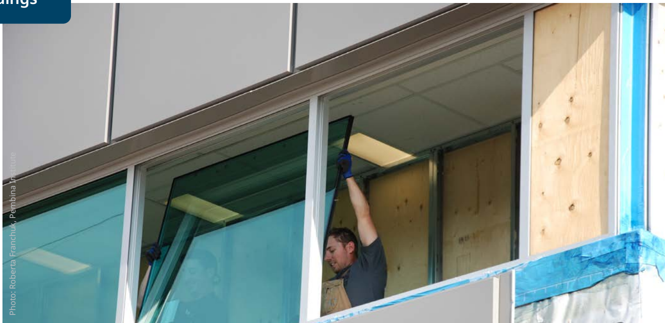
Energy retrofit of commercial building
