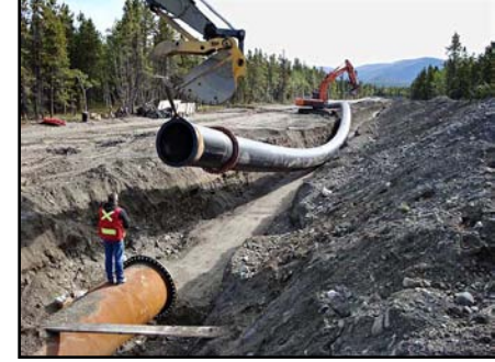
Atlin, BC Project Installation
