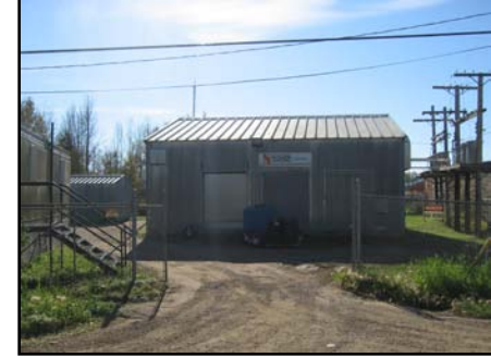
Power Station Fort Liard, NWT
