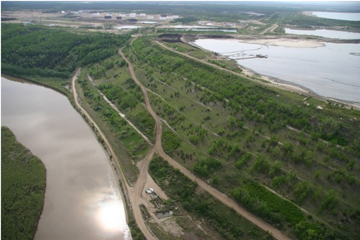
Figure 10 Suncor's Tar Island Dyke (center of the photo) separates an oil sands tailings pond (upper right) from the Athabasca River.
