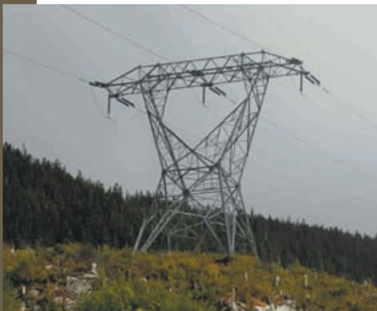
A 287-kV transmission line from Kemano to Kitimat in British Columbia.
