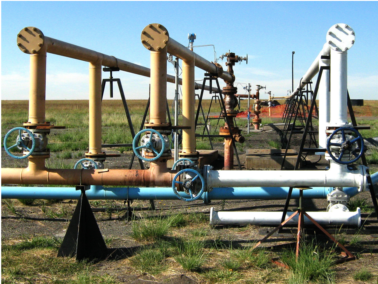
▲ Ergo Exergy's Operating Underground Gasifier, surface pipeworks, 2009.
