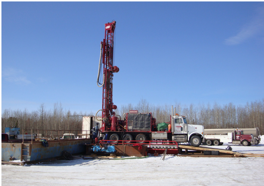
▲ Hydrogeology investigation (pumping well drilling) at a UCG site in Alberta, 2009. Courtesy of Laurus Energy Canada
