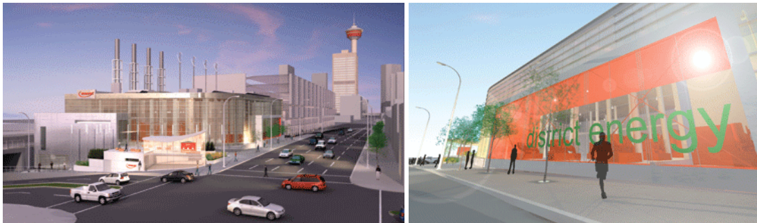
Figure 27. ENMAX is currently constructing a district energy plant in downtown Calgary to provide heat to the surrounding buildings. There are plans to eventually turn it into a cogeneration plant using waste heat from an electricity generator.
