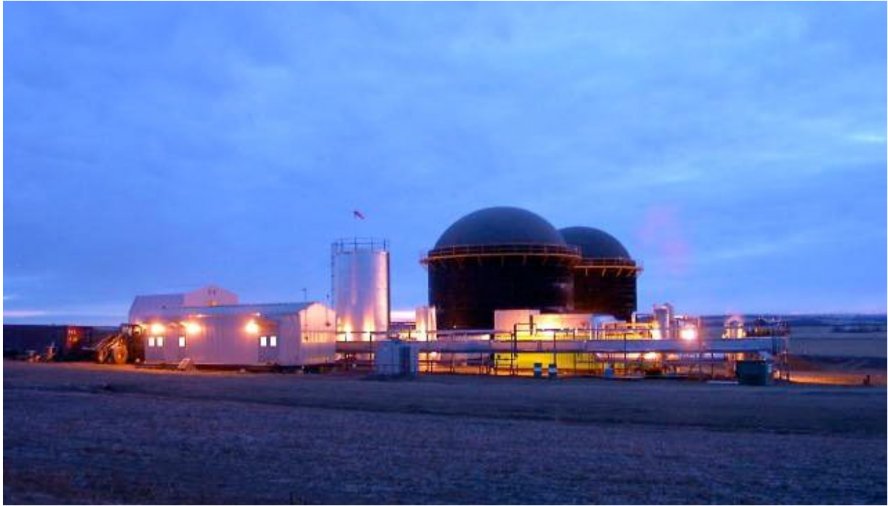
Figure 23. The Integrated Manure Utilization System in Vegreville, Alberta, generates electricity and uses waste heat for internal processes
