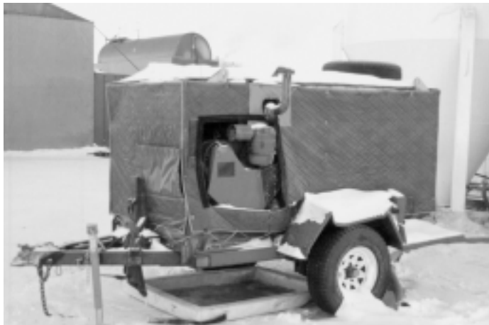
Drip tray to prevent soil and water contamination
