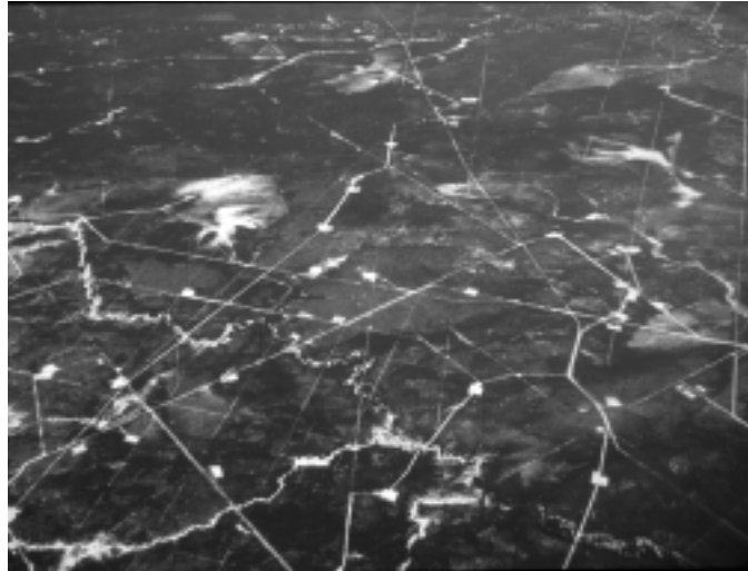
Well pads and roads near Grande Prairie Alberta.
