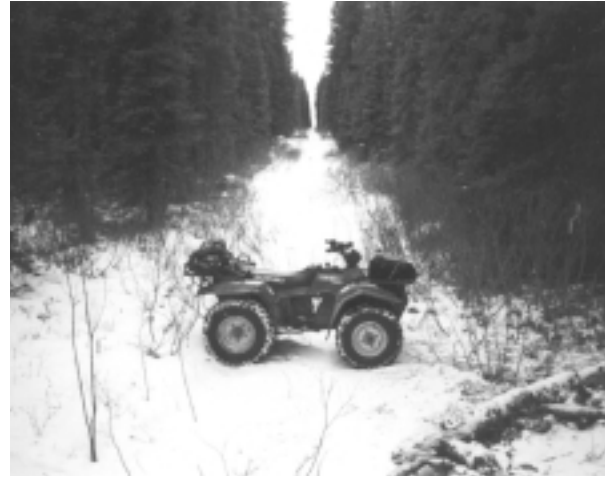
A mechanically cut, high-impact seismic line, six metres wide.
