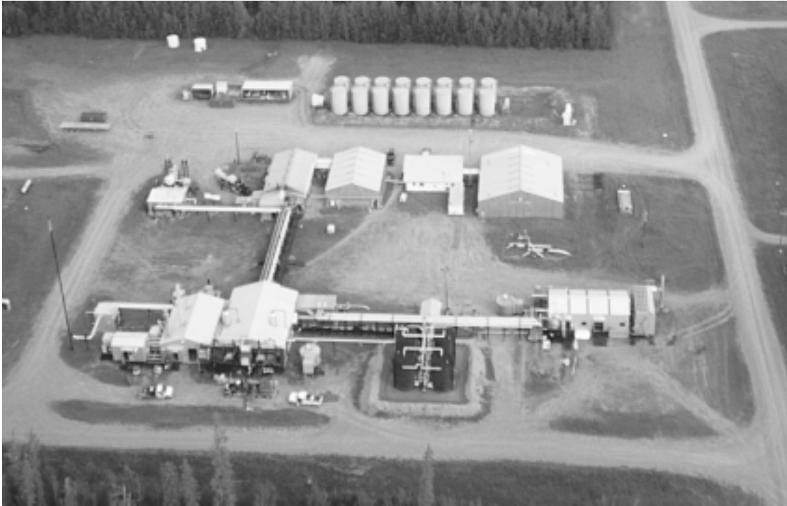
West Coast Pine River Gas Plant BC
