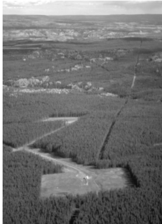
Wellpad and a Right of Way in the Sikanni. Regulators could require companies to share the use of roads to avoid more roads in the area.
