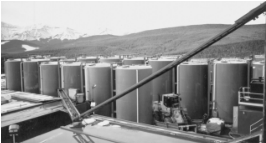
Storage tanks for storing drilling waste
