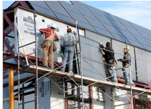
Figure 2: CLEAN contracts can be developed for both solar photovoltaic and solar hot water systems (Photo: Gordon Howell).
