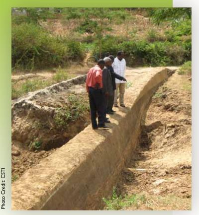
Sand dams constructed in Sakai and other parts of Kenya have proven to be reliable sources of water for people, livestock and plants during the dry season and in times of drought. By slowing the flow of creeks or rivers, these dams trap sand (which prevents evaporation) and cause water to percolate underground, where it remains available for future use.
