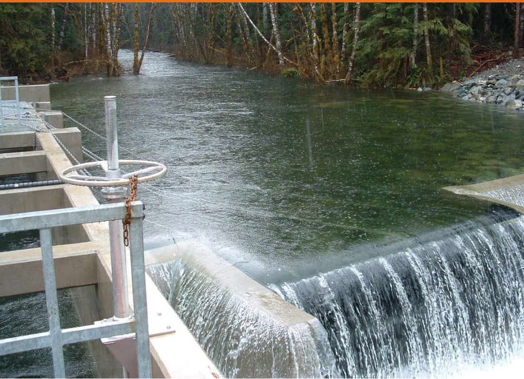
The China Creek run-of-river project completed by the Hupacasath First Nation near Port Alberni, British Columbia.
