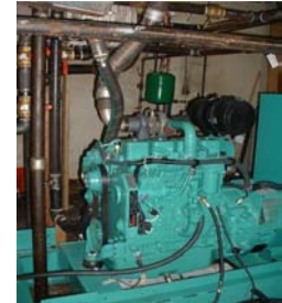
The coolant from diesel engines can be used to heat nearby buildings.
