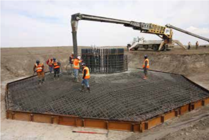
Workers undertaking the cement pour on a turbine foundation. A single foundation may include 44 tonnes of rebar and require 40 truckloads of cement.
