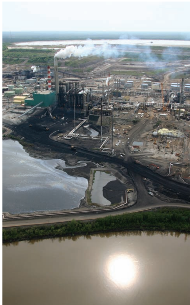
The Suncor Oil Sands complex along the Athabasca River north of Fort McMurray. Photo: David Dodge, The Pembina Institute
