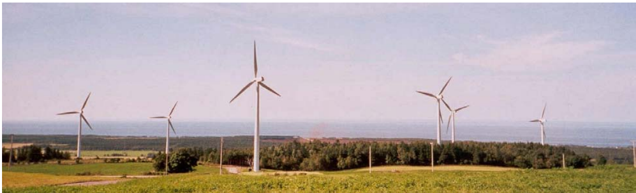
Figure 4.3 Wind power is an abundant source of renewable energy
