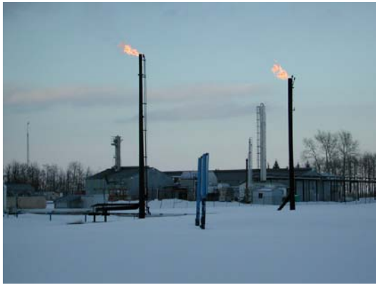
Figure 2.4 Gas flare at a compressor station in Drayton Valley
