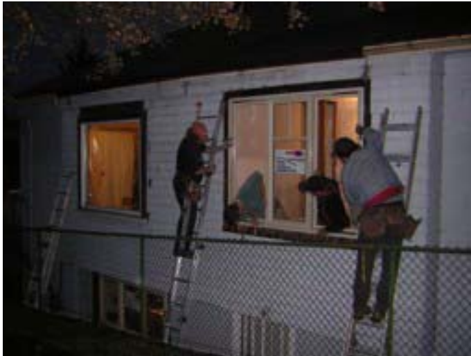
Figure 4.6 Installing new windows in a home is one means of improving energy efficiency
