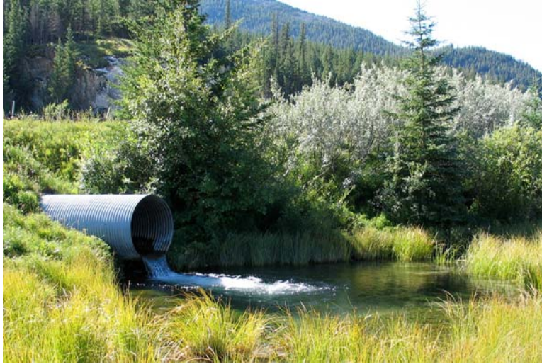
Figure 3.4 Hanging culverts prevent fish movement upstream
