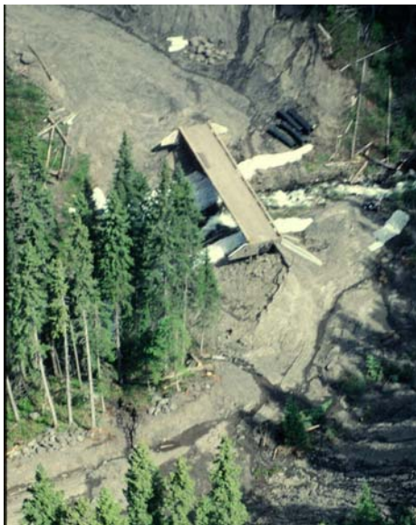
Figure 3.5 Road washing out into streambed in northeast British Columbia
