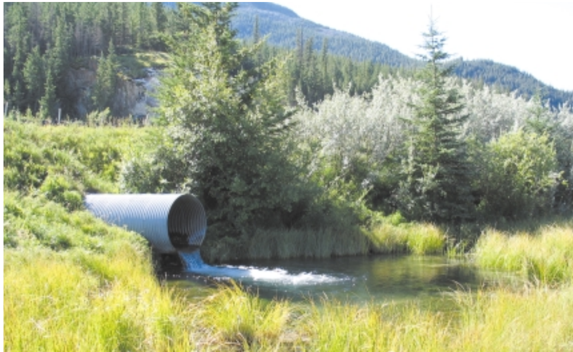
▲ Hanging culverts prevent fish movement upstream.
