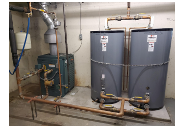
Natural Gas DHW Boiler Storage Tanks
