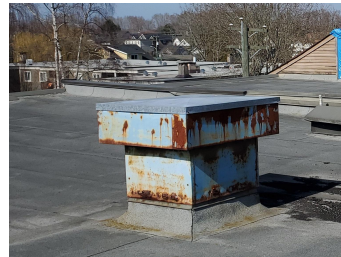
Unheated Rooftop Fans Corridor Ventilation
