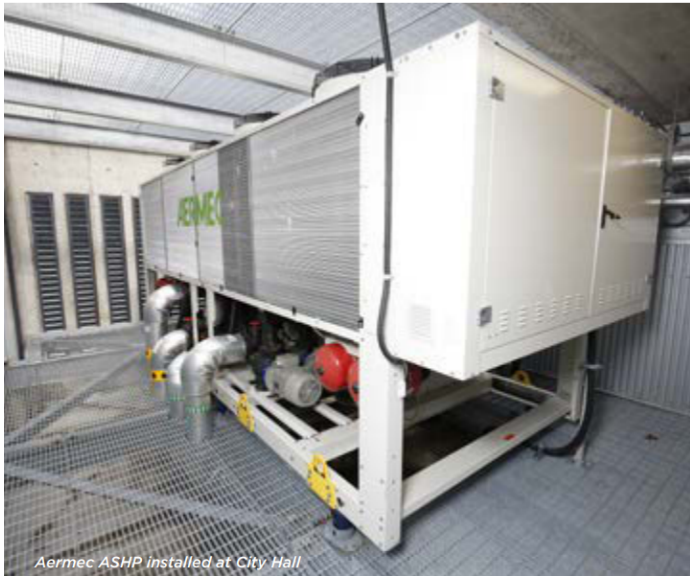
Aermec ASHP installed at City Hall
