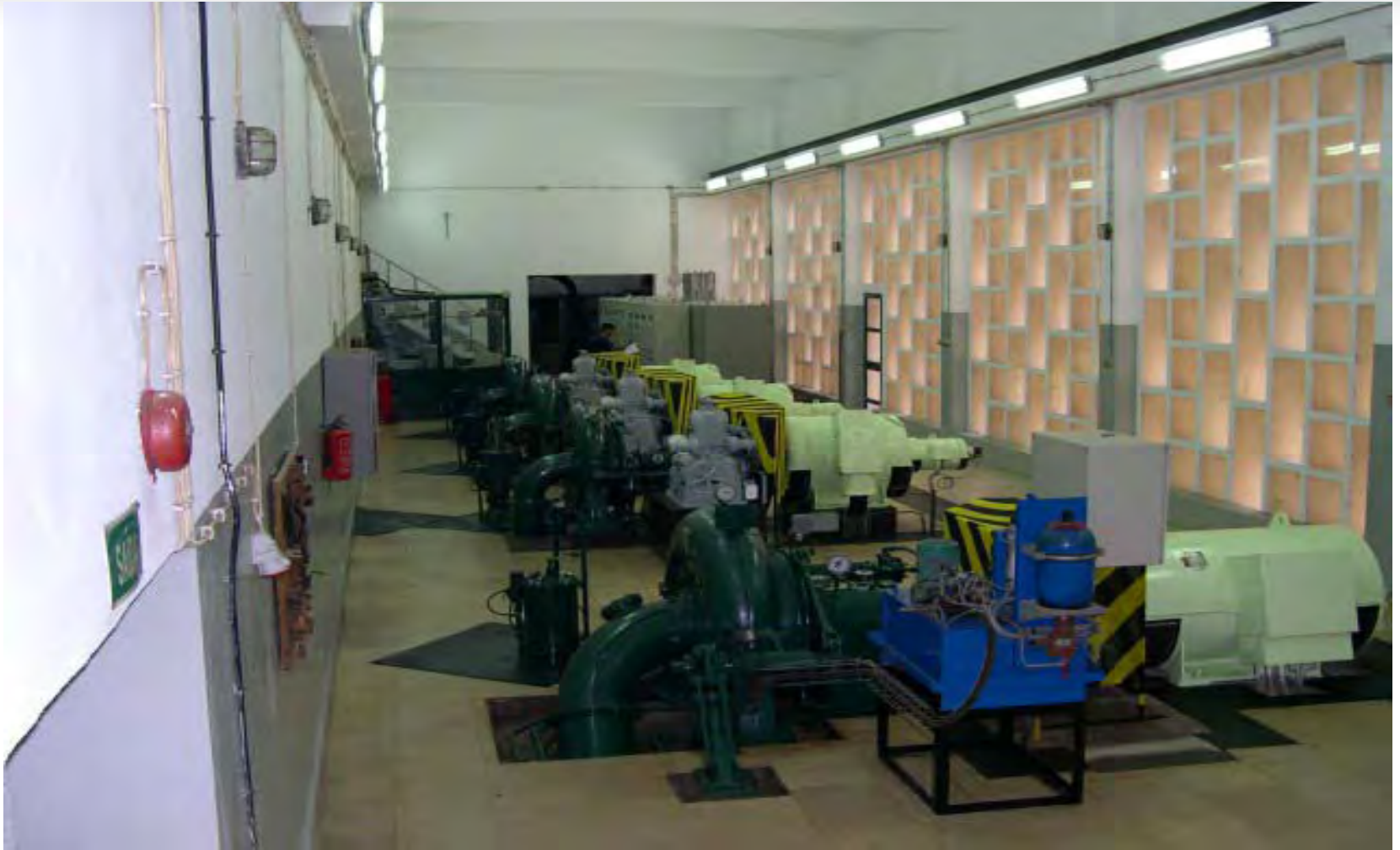
Combined hydro (1,100kW) and diesel power station (4,000kW)
