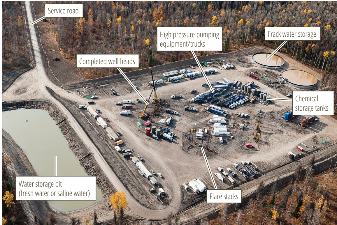
Figure 4. Hydraulic fracturing site
