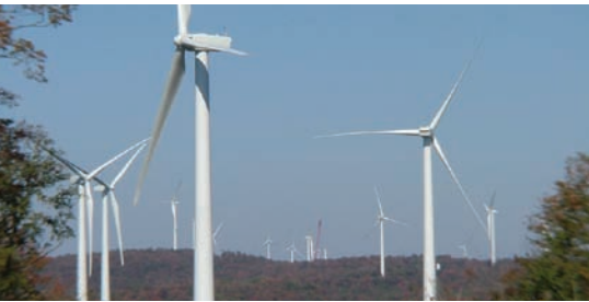
This wind farm near Sault Ste. Marie was built on-time and on-budget, and now provides enough power for 40,000 homes.
