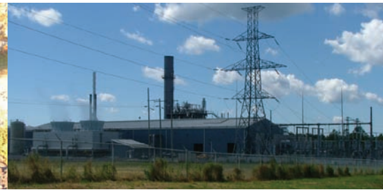
This cogeneration plant near Kingston uses a waste energy recycling process to produce both electricity and industrial steam for adjacent industries.
