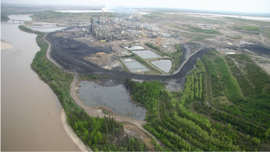
Figure 22: The long-term viability of tailings dykes will remain an ongoing concern long after operations cease. Dyke failures could release unstable materials into the Athabasca River, with catastrophic effects on the aquatic ecosystem.
