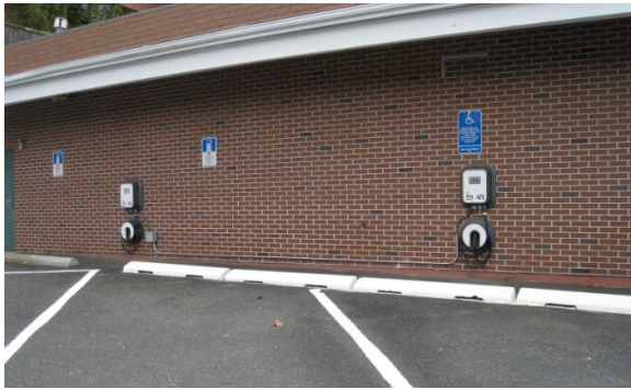
Two Level 2 wall-mounted charging stations at a city-owned public parking lot in Lake Oswego. Source: City of Lake Oswego, 2012.
