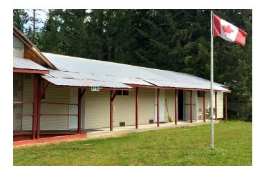
The Seniors' Centre is a small, single-story 1,200-ft<sup>2</sup> wood-framed structure that consists of a meeting place, library, kitchen and washrooms. It was built in 1977 using standard construction techniques, and the exterior has mainly remained unchanged.
