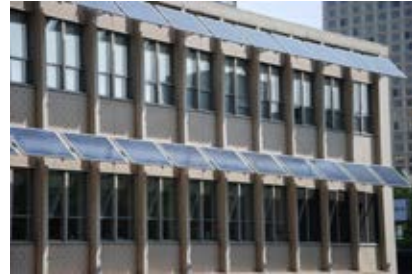
Solar panels have higher net costs but the price of technology continues to drop.
