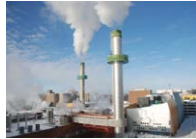
Distributed energy systems are used in some parts of the city, including the University of Alberta.
