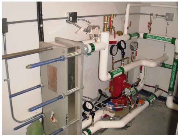
Langley's geoexchange heating system. Source: Township of Langley.
