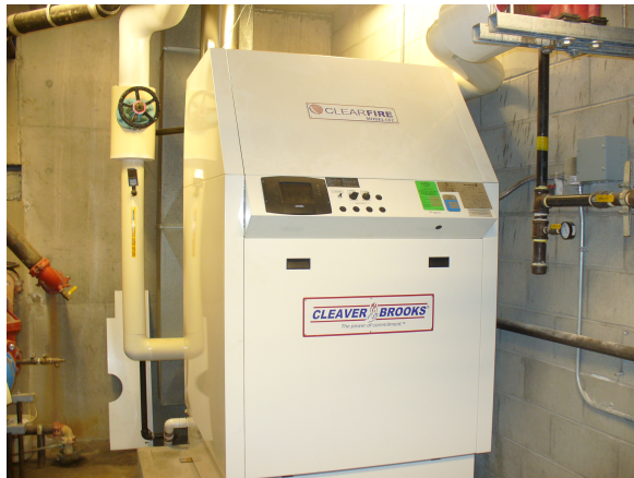
Cleaver Brooks Clearfire condensing boiler. Source: Corporation of Delta.
