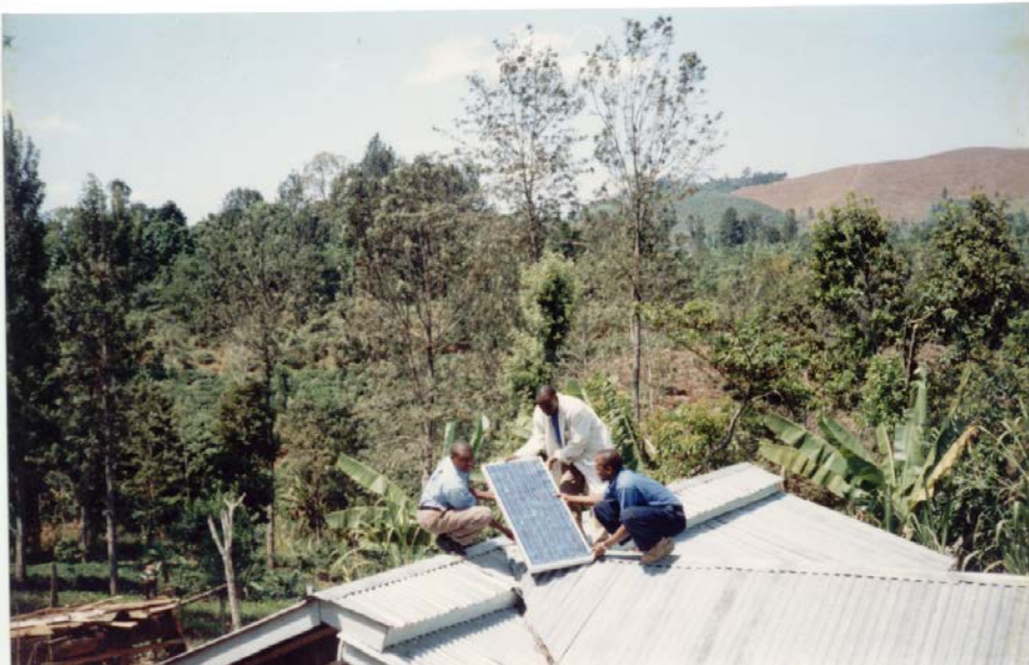
Technicians Installing a Domestic Solar System in Rural Kenya
