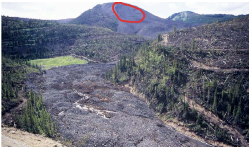
More than 60,000 cubic metres of rocks traveled two kilometres in less than one minute when a waste rock pile at a Southeast British Columbia mine collapsed. The pile's original location is shown in the background of this photo. PHOTO: O. HUNGR
