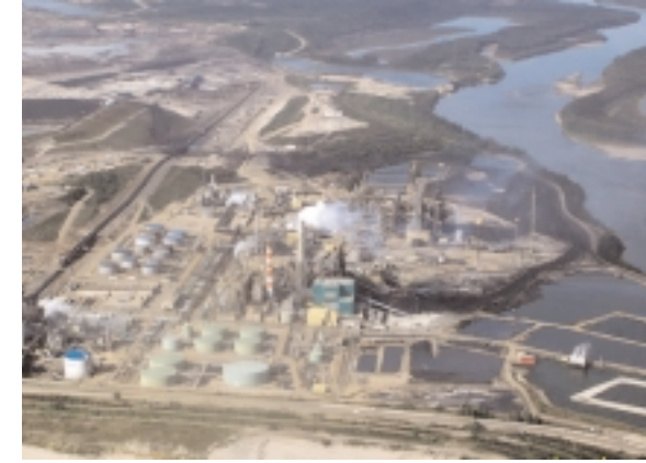
▲ Oil sands upgrader plant and related facilities. PHOTO: CHRIS EVANS
