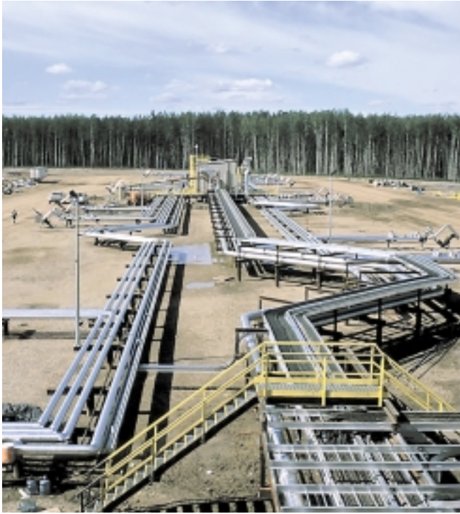
▲ FIGURE 2 (photo above): Pipeline gathering system in a SAGD installation.
