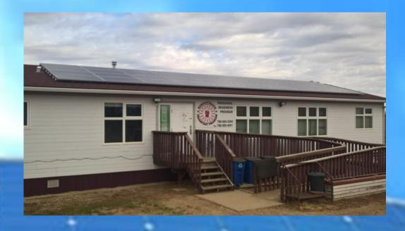
10 KW - 40 Solar PV modules at 255 watts each 20 - 500 watt APSystem Dual Micro-Inverters
