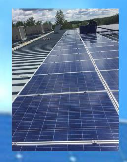
40 KW - 160 Solar PV modules at 255 watts each 80 - 500 watt APSystem Dual Micro-Inverters
