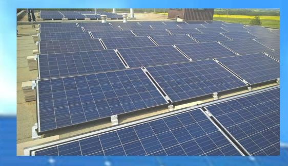
25 KW - 100 solar PV modules at 260 watts each
